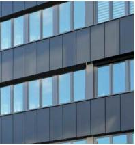
50-year-old building was completely renovated, technically and energetically brought up to date according to Energy Efficiency 100. 234 anthracite-colored SKALA modules were integrated into the facade below the window strips and on the parapets. integrated into the facade.
