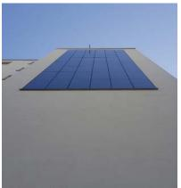
As part of a modernization project, the 36 houses implemented an energy concept consisting of combined heat and power units and renewable electricity from photovoltaic modules was implemented. The 100 square meter photovoltaic system blends harmoniously into the overall appearance of the building.
