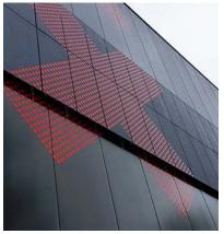
Solar facade with grey SKALA modules on the south and west side of the new depot of the Amsterdam City Archives. A total of 800 rooftop PV modules and 300 modules on the facades ensure the yearly energy self-consumption of the new energy efficient building.
