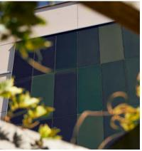
The building envelope of the residential complex was totally refurbished with penthouse apartments. The property rated with an energy efficiency label AA+ generates electricity and hot water via PV modules on the roof, on balcony parapets as well as two SKALA solar facades.
