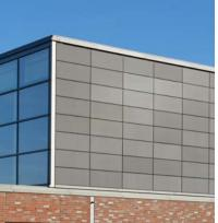
At the new three-field sports hall of the comprehensive school in Gronau, 536 anthracite-colored SKALA modules on three sides of the upper floor provide a visual contrast to the red clinker facade on the first floor for sustainable power generation.
