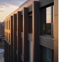
Seven storey office building in new wood-concrete hybrid construction with mixed use of office space, medical practices and other services. The cladding material of the energy efficiency house is a solar facade made out of bronze SKALA modules.
