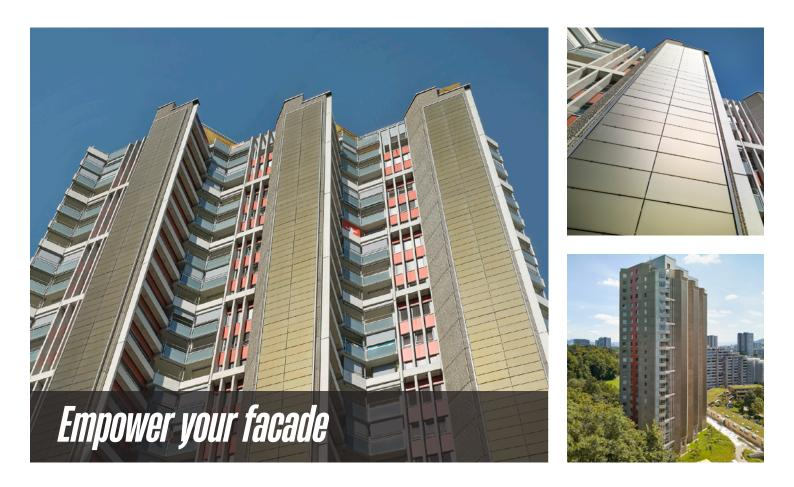
In this Swiss pilot project regarding fire protection regulations, a solar facade with a special substructure was integrated into the building envelope as part of a refurbishment of 54 m high concrete facade strips on two high-rise buildings.
