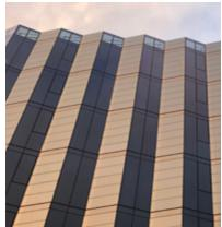
On Australia's first solar facade, transparent window surfaces were combined with opaque solar modules consisting of light grey SKALA modules. The elements made of different facade materials were installed that they are optimally orientated the solar radiation.
