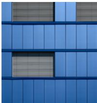
The energy-efficient refurbishment was carried out during ongoing operations. In addition to the roof-mounted PV systems, the west side was given a solar facade in the customer color "Volgblau" with standard and reduced-length modules.
