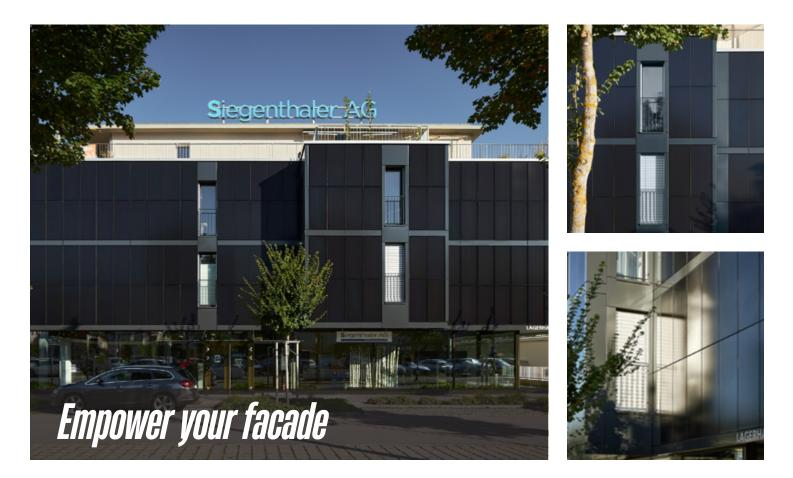
New construction of the energy-efficient residential and commercial building with a solar facade on the south-east side of the building. Our black frameless SKALA modules meet all the requirements for aesthetics and high quality.
