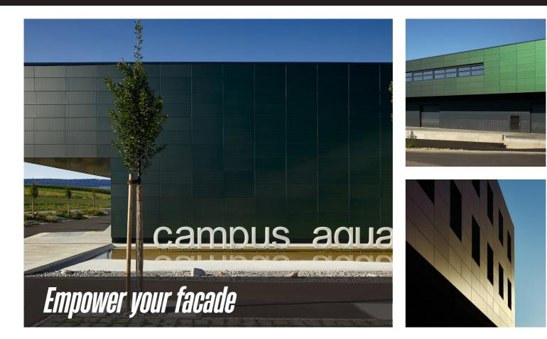
New warehouse surrounded by a complete solar facade mounted on the north, east, south and west facade. The solar facade is composed of green SKALA modules in standard size combined with customized lengths covering 70 % of the energy self-consumption of the building.
