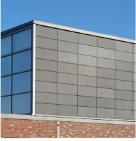
At the new three-field sports hall of the comprehensive school in Gronau, 536 anthracite-colored SKALA modules on three sides of the upper floor provide a visual contrast to the red clinker facade on the first floor for sustainable power generation.
