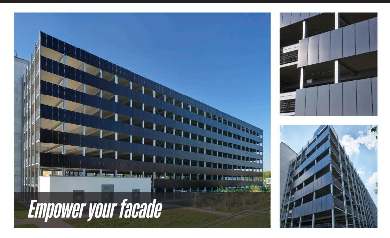
The use of a simplified substructure makes the realisation of the solar facade on this multi-storey car parking house particularly attractive and is therefore groundbreaking for the further development installation use on industrial facades.
