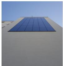
As part of a modernization project, an energy concept consisting of combined heat and power units and renewable electricity from photovoltaic modules was implemented in 36 houses, each with a 100 m<sup>2</sup> facade system consisting of black SKALA modules.
