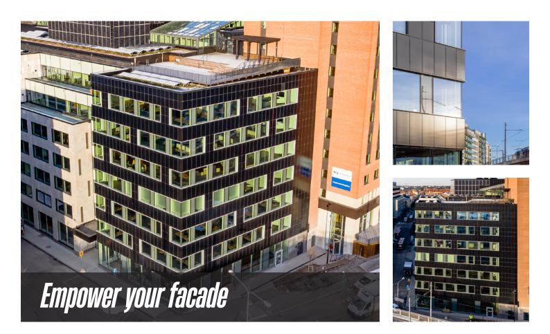
As part of an extension, the office building was designed to achieve the highest level of LEED Platinum Core & Shell environmental certification. The black SKALA modules integrated between the ribbon windows play a part in this.
