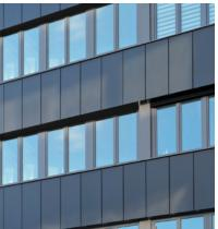
50-year-old building was completely renovated, technically and energetically brought up to date according to Energy Efficiency 100. 234 anthracite-colored SKALA modules were integrated into the facade below the window strips and on the parapets.
