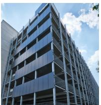
The use of a simplified substructure makes the realisation of the solar facade on this multi-storey car parking house particularly attractive and is therefore groundbreaking for the further development installation use on industrial facades.
