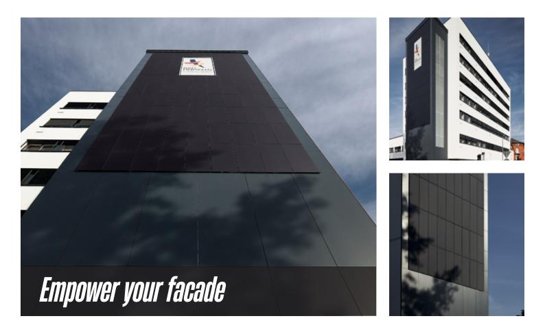
During the renovation of the Stadtwerke Bad Hersfeld high-rise building, the south-east side was extended with a solar facade consisting of anthracite-colored SKALA modules and thus upgraded to an energy-efficient facade.
