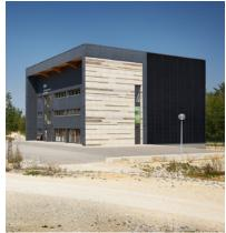
Construction of a modern climbing center of the German Alpine Club with a 169 m<sup>2</sup> large solar facade on a wooden substructure on the south side of the envelope. The JURABLOC impresses with the unique combination from natural stone facade and different materials.
