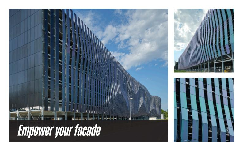
In our first hybrid project, the new parking garage of DHL, building-integrated photovoltaics in the building envelope and rooftop solar systems were combined to cover a large part of the DHL campus' electricity requirements.
