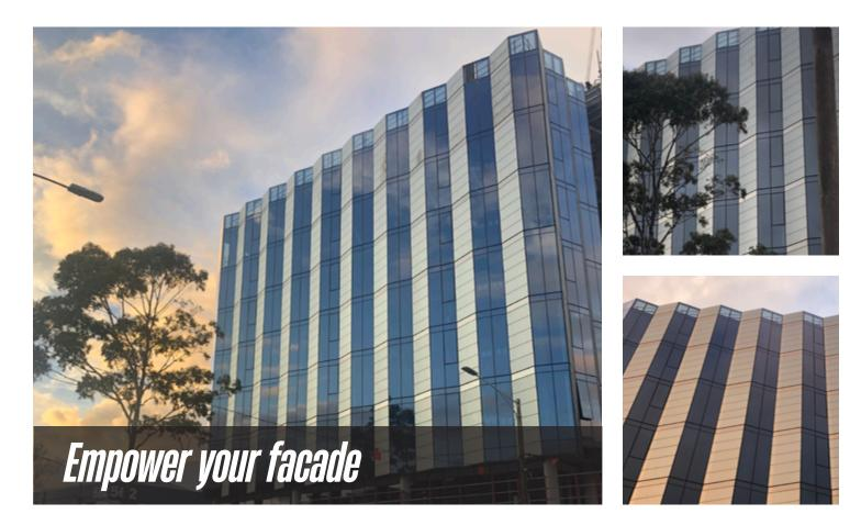
On Australia's first solar facade, transparent window surfaces were combined with opaque solar modules consisting of light grey SKALA modules. The elements made of different facade materials were installed that they are optimally orientated the solar radiation.
