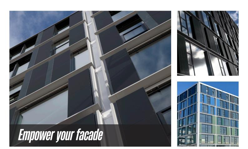
This multifunctional building for the University of Amsterdam is designed to be flexible, sustainable and demountable. The modular facade construction combines colored ceramic elements with anthracite-colored SKALA modules.
